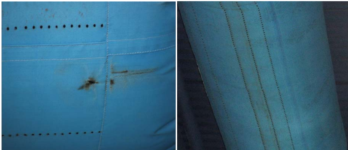
Figure 7: Accumulation of dust - textile sheaths
